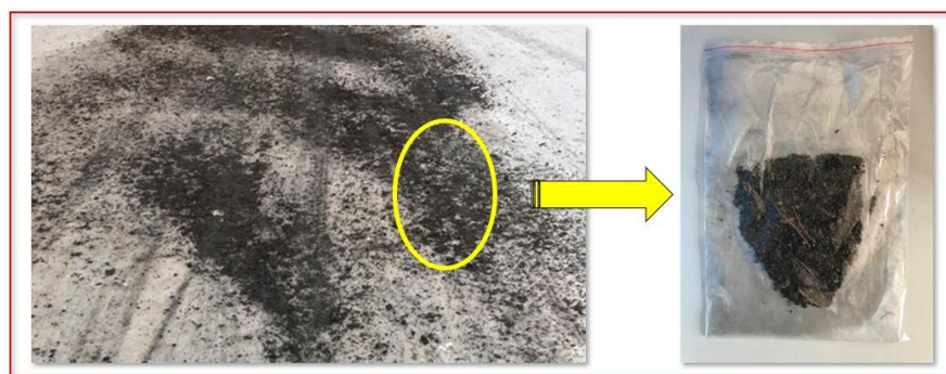
Figure 3. Anti-slip sand thrown on permeable pavement.
