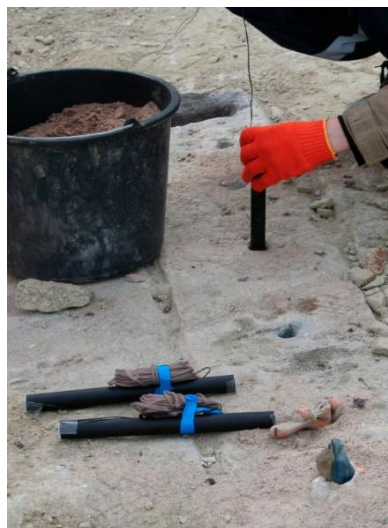
Figure 8. RSP, and the method of its insertion into the blasting hole.
